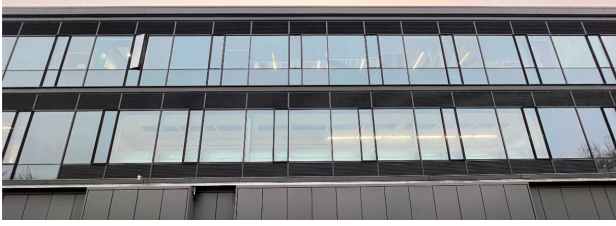
(a) Picture of the building façade
