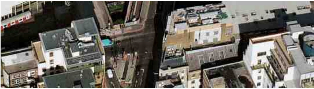
546. Clerkenwell Road, looking east from Farringdon Road, in 2001. Metropolitan Railway cutting and Vine Street Bridge in foreground
