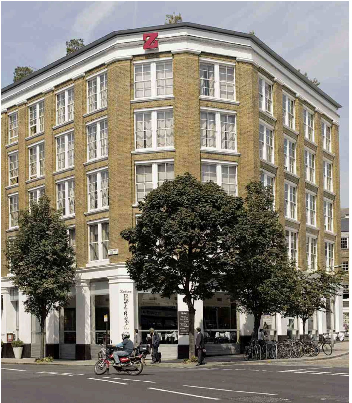
553. Nos 86–88 in 2006; warehouses of 1884–6 (now The Zetter hotel)
