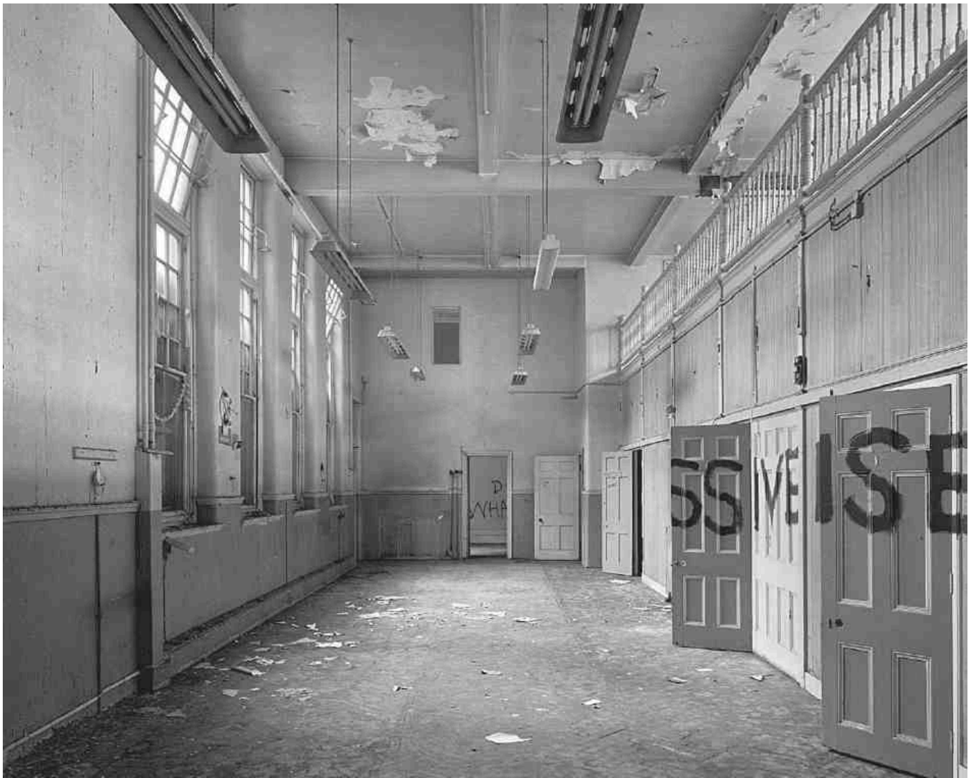
564, 565. Nos 49–53 Clerkenwell Road, interiors in 1993. The former boardroom and (right) outpatients' waiting-hall and examination rooms
