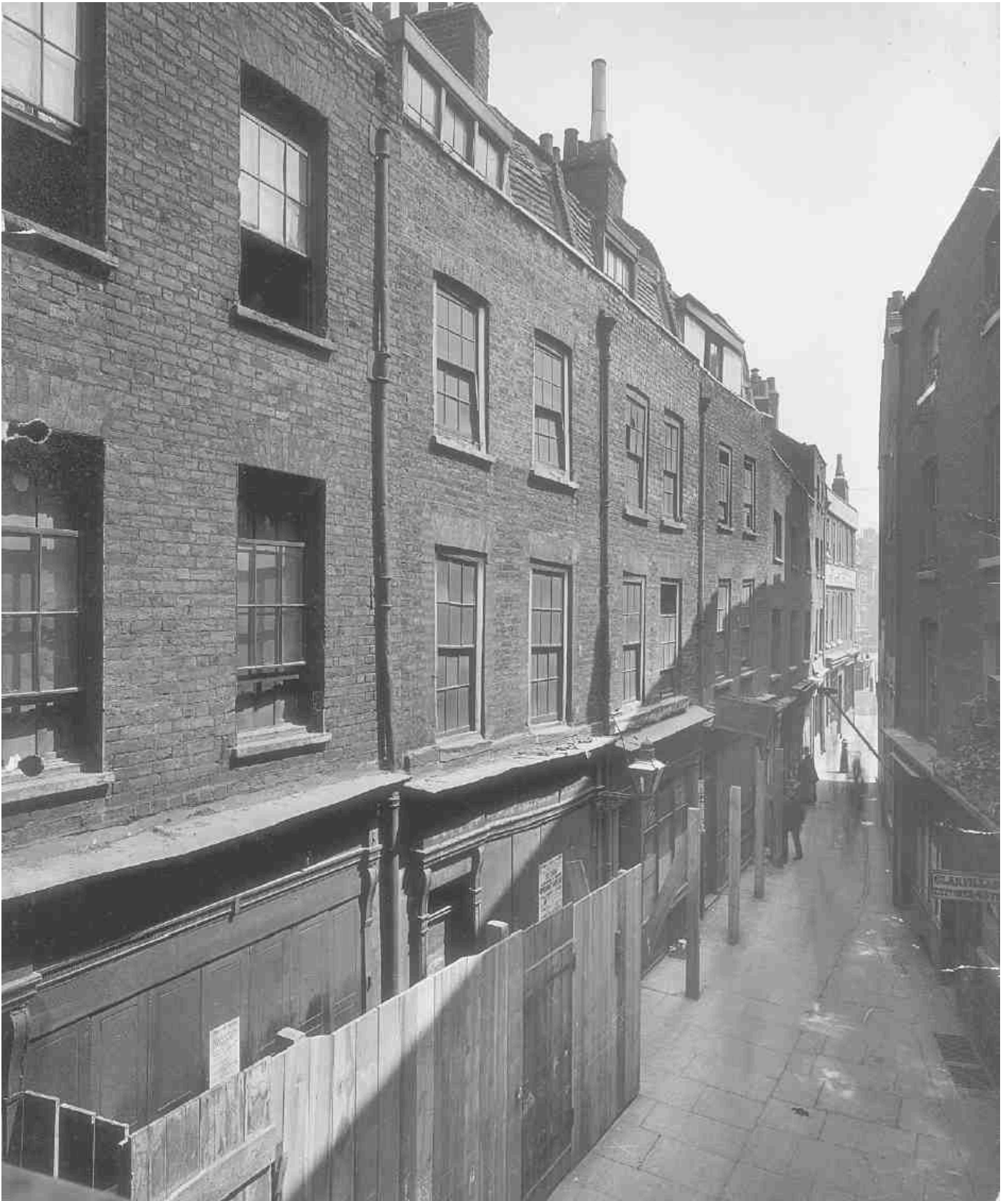
138. Jerusalem Passage, east side, in 1906. Foreground: houses of the 1720s at Nos 1–4, shortly before demolition
