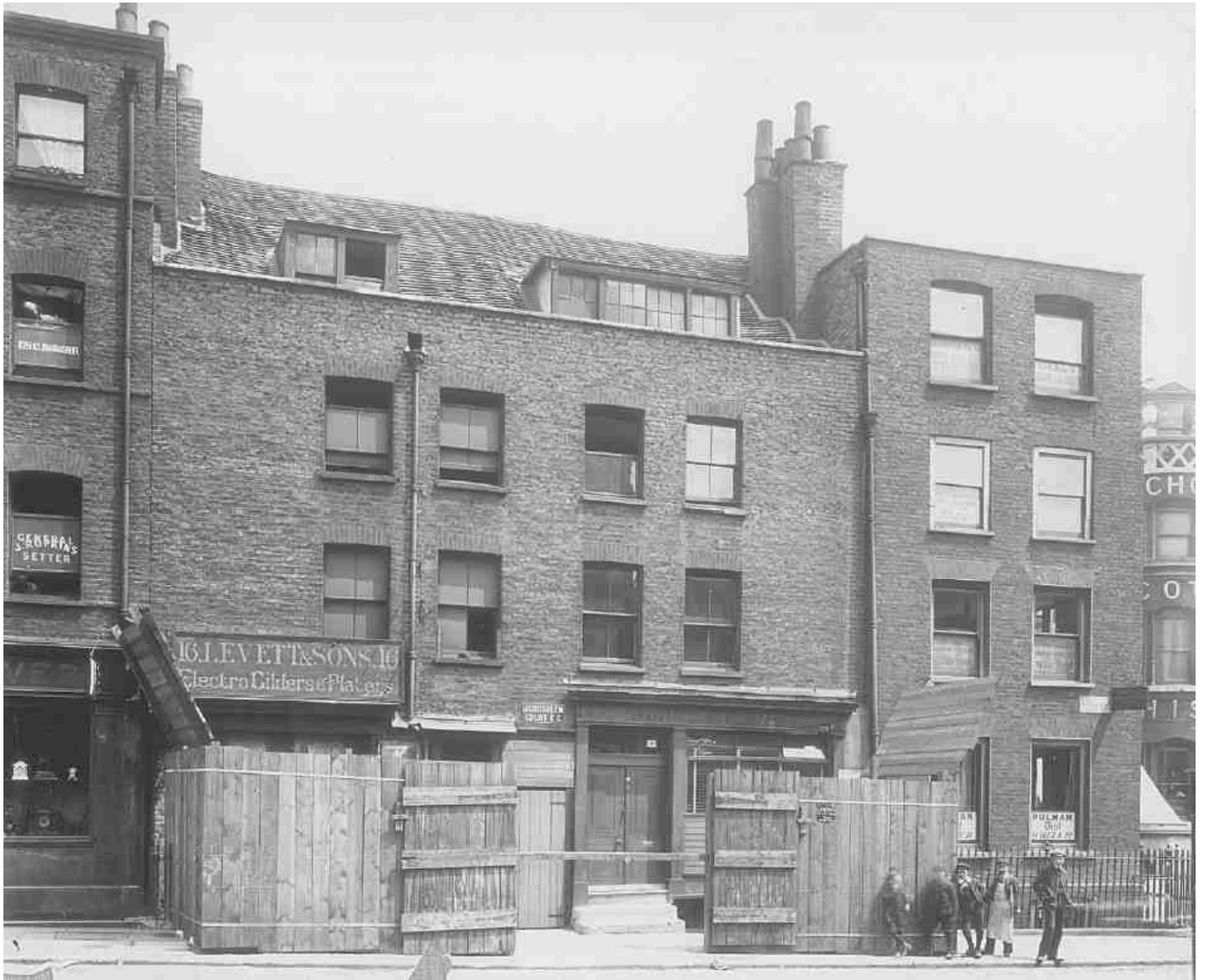
139 (top right). Nos 15 and 16 St John's Square, of c. 1692, photographed in 1906. Demolished
