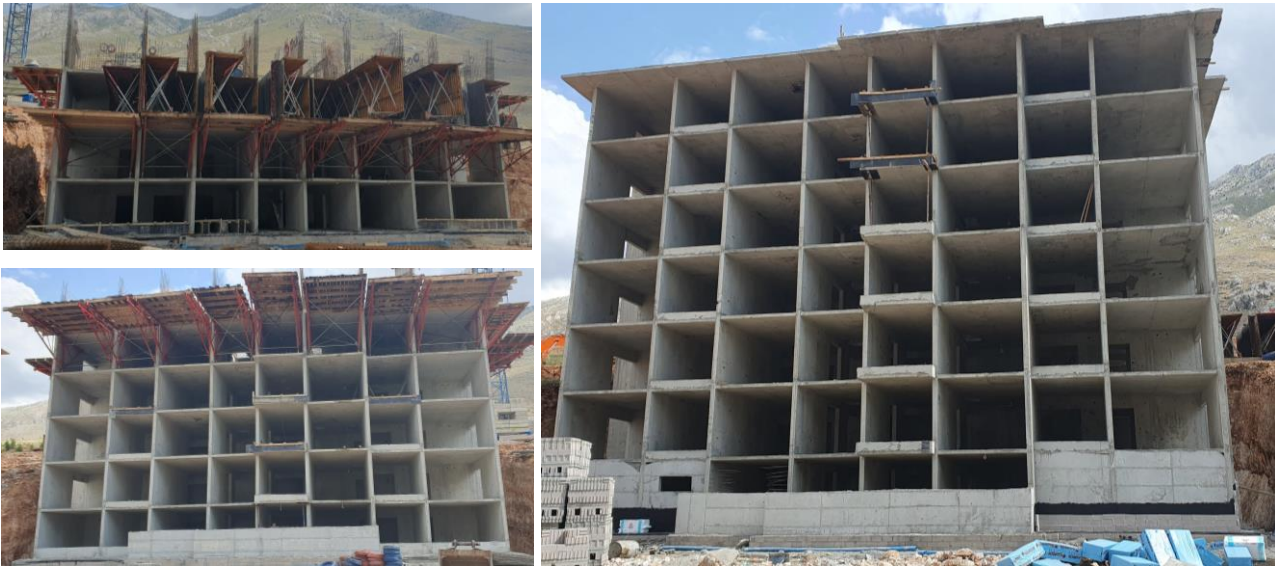
Figure 1. Tunnel-formwork application.
