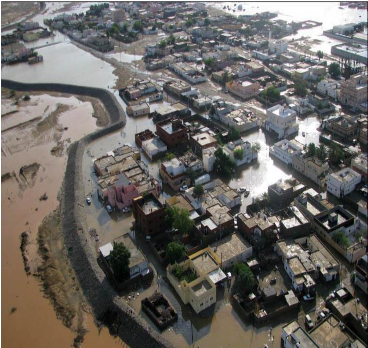
Figure 2.3. Flood of Jeddah – November 2009 (Azeez et al., 2020)
