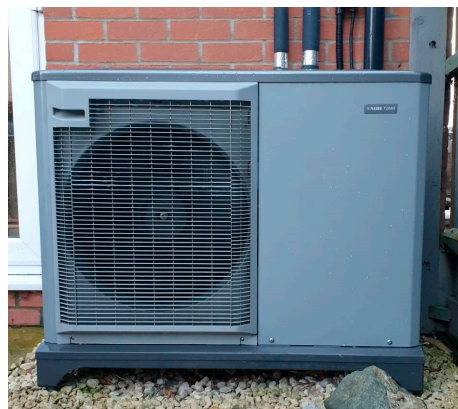
Figure 1. Typical UK domestic heat pump outdoor unit.
