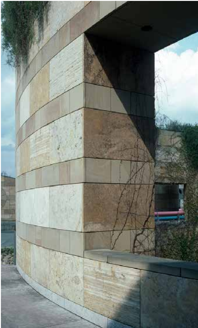
8 James Stirling, Staatsgalerie, detail of cladding in sandstone and marble, 1977–1984, Stuttgart
