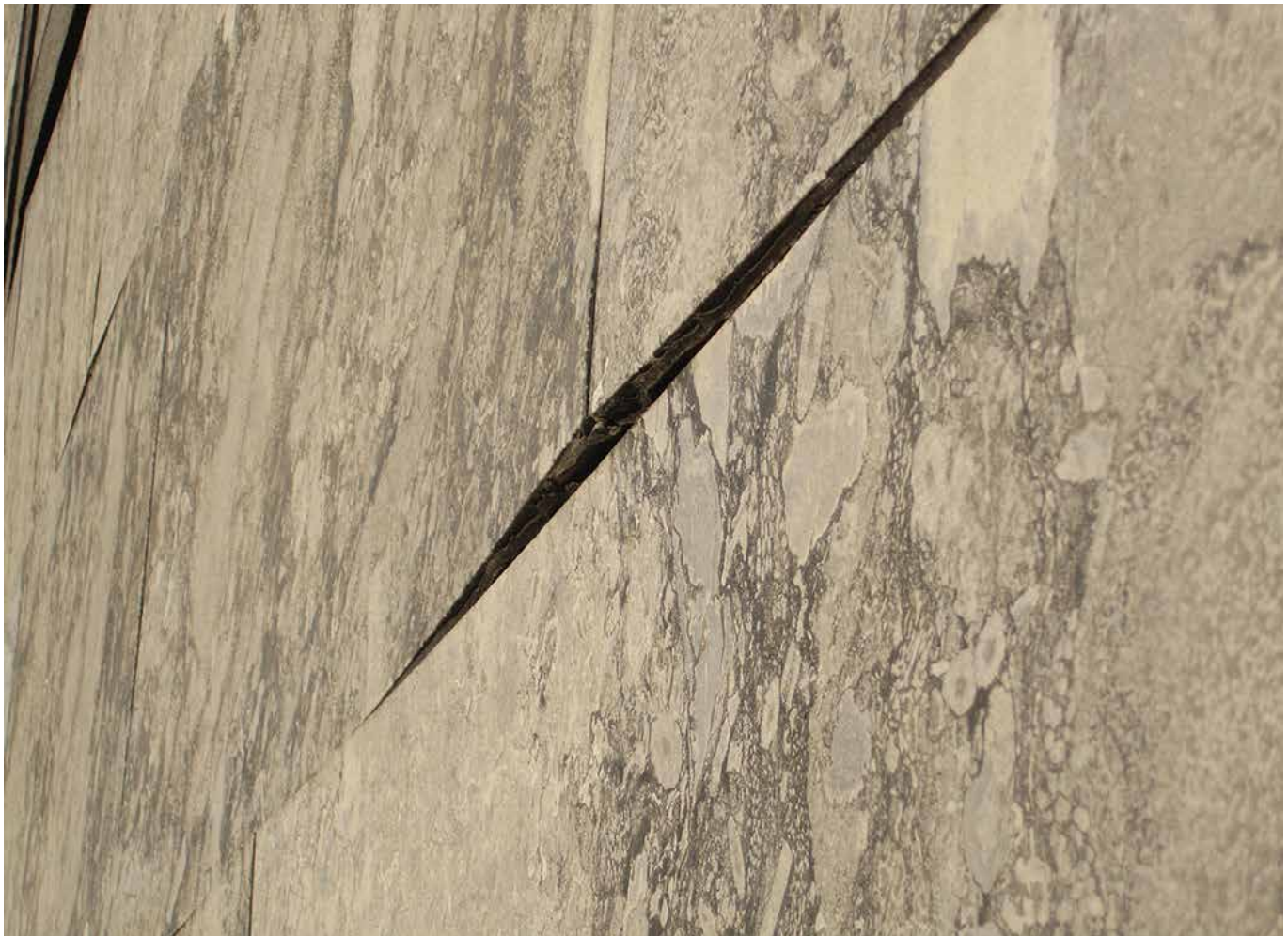
6 Arne Jacobsen, Danish National Bank, Copenhagen, 1965–1978, detail of deformed Porsgrunn marble revetment, photographed in 2017
