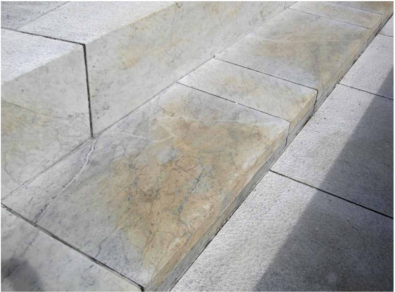
11 Snøhetta, Opera House, 2000–2008, Oslo, detail of Carrara marble paving showing staining, photographed in 2016
