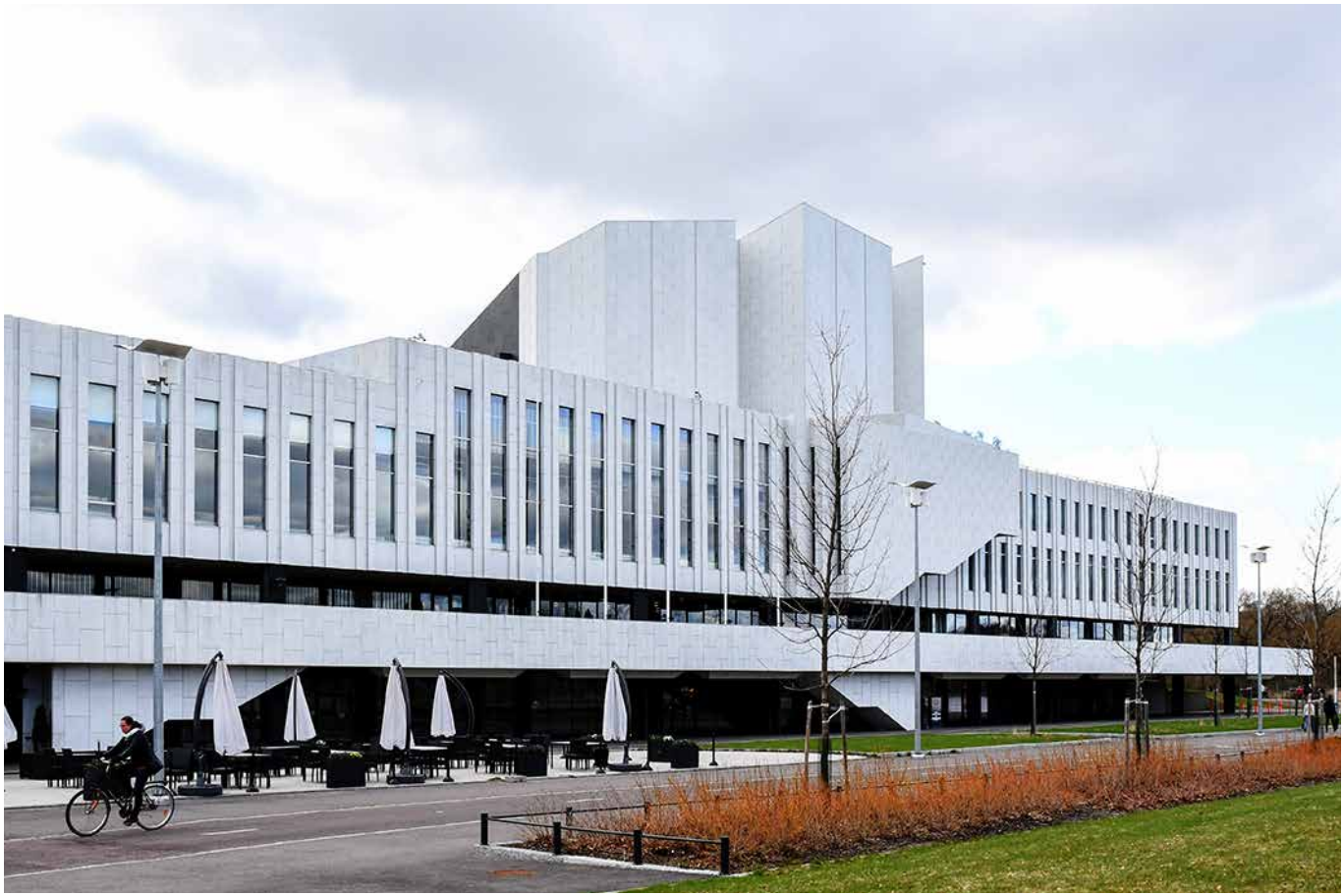
3 Alvar Aalto, Finlandia Hall, 1967–1972, Helsinki, after 1997–1999 recladding with Carrara marble, photographed in 2018
