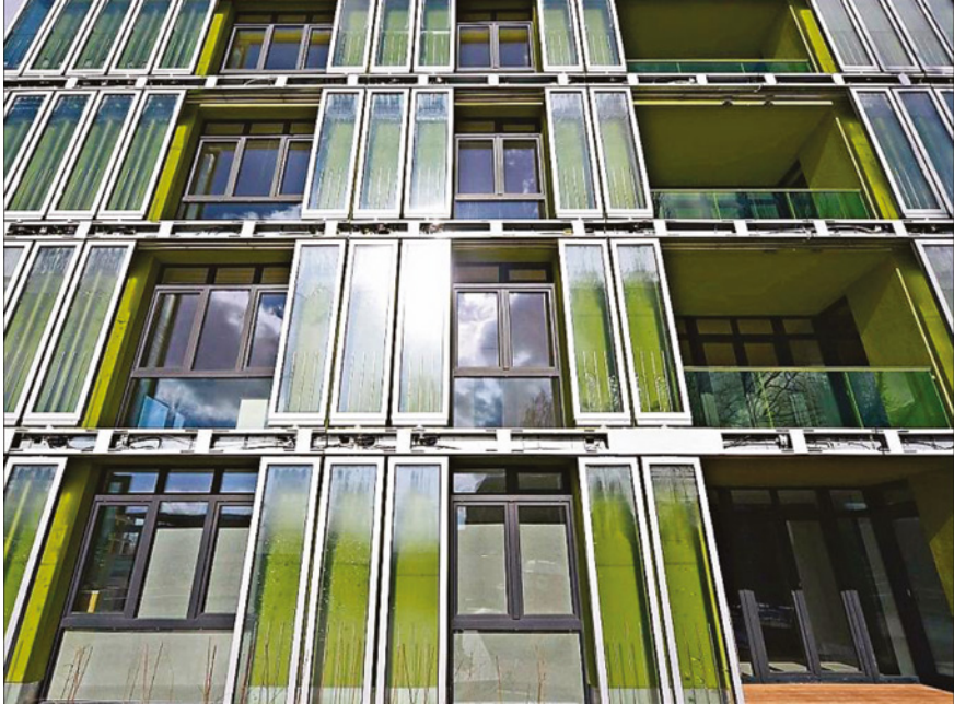
FIGURE 11.1 Solarleaf façade of B.I.Q. House with algae monoculture in flat bioreactors built on the occasion of the International Building Exhibition in Hamburg, 2013. Team: ARUP Engineering in collaboration with the Strategic Science Consult and Colt International PHOTO CREDIT: MARCOS CRUZ
