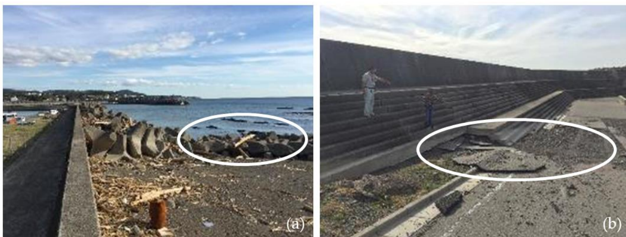
Figure 2. a) Displacement of artificial armour units, and b) damage to the landward toe of the seawall in Inami Town due to Typhoon 24 in 2018 (white circles indicate the damage).
