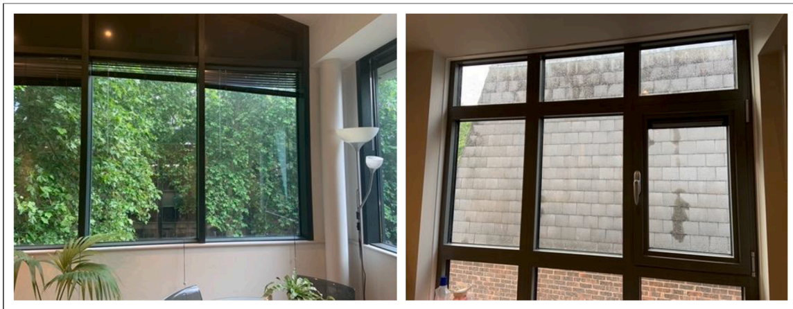
Fig. 5. LEFT: Resident experiences overheating as only the window on the far right opens. RIGHT: Resident could not install barrier to light on the large window and it did not open upon occupation of the flat.
