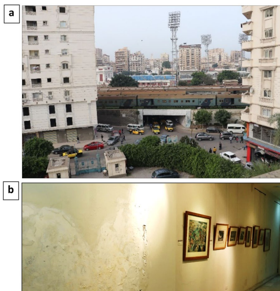
Fig. 3 a shows the museum entrance near the train station, tunnel, stadium, adjunct high buildings; b shows the salt weathering and dampness in the wall behind the painting
