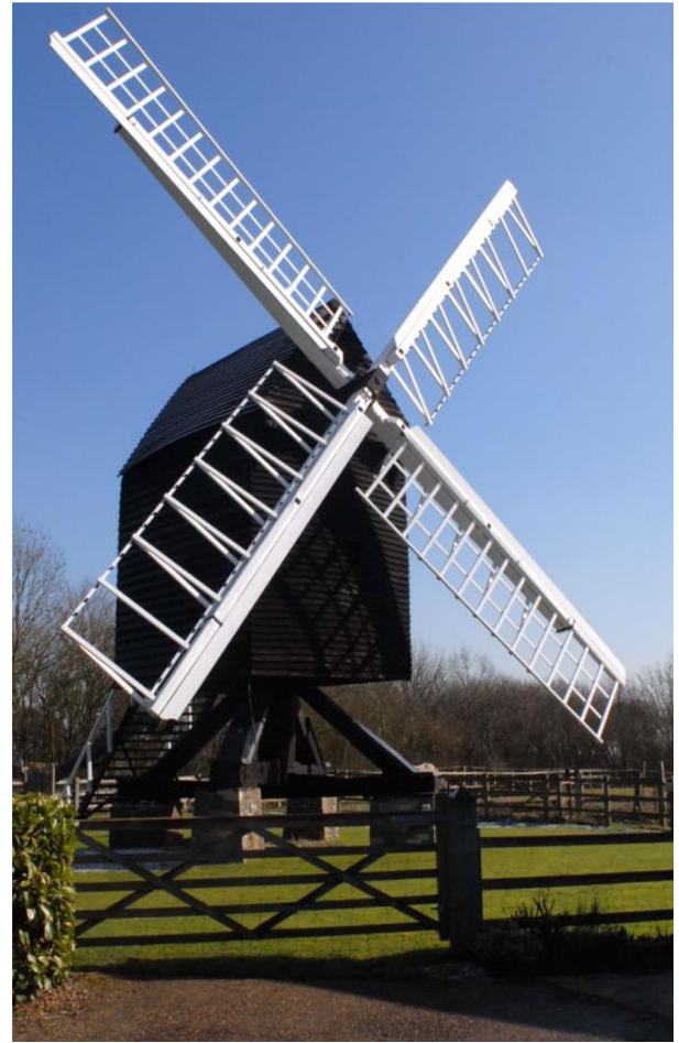
Figure 2. Bourn Windmill (Cambridgeshire). Note the open trestle supported on brick plinths, pitched roof shape and two plain sails (photo: Martin Davies)
