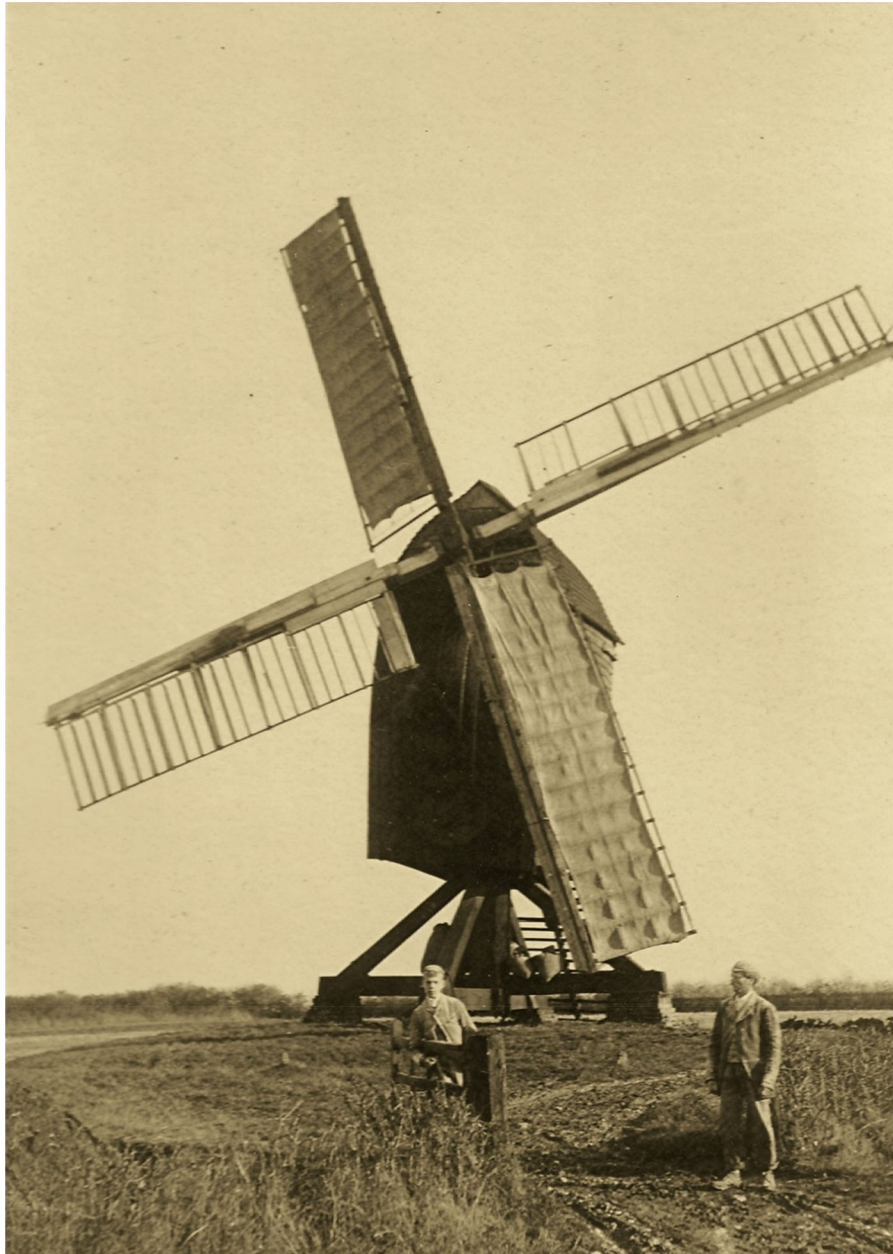
Figure 3. Gransden Windmill in its working days in the early 1870s—a rare early photograph of a typical early post mill. Note the open trestle supported on brick plinths, the two plain sails with cloths unfurled and the curved roof shape (photo: Revd Frederick Le Grice. From Gransden Society Archives)
