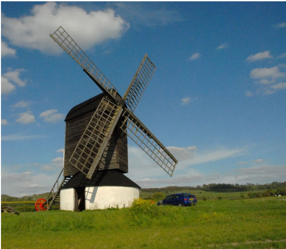
Figure 9. Pitstone Windmill (Buckinghamshire). Note the full set of four plain (cloth) sails (photo: Martin Davies)
