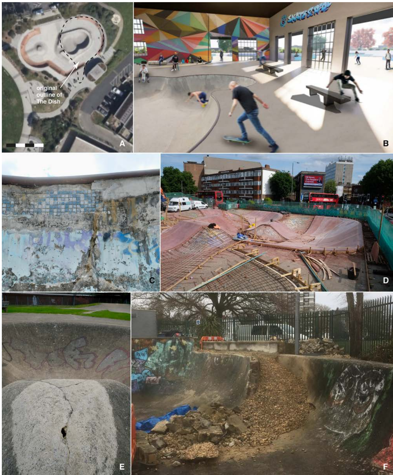
FIGURE 10. Preservation, repair and conservation of heritage skateparks. A. ‘Renovation’ of The Dish, San Francisco with footprint of the original bowl. Source: DuckDuckGo maps. B. Artist’s impression of the planned restoration of The Turf, Milwaukee. Source: School of Architecture, University of Wisconsin-Milwaukee. C. Close-up of degraded and poorly repaired Pool Bowl at Solid Surf, UK. Photographer: Patrick Quinn. D. Re-surfacing of Stockwell, UK in summer 2022. Photographer: Patrick Quinn. E. Polished concrete test area at Solid Surf. Photographer: Patrick Quinn. F. Removal of historic ‘improvements’ to the Spoon Bowl at Southsea Skatepark, UK in 2018. Photographer: Sam Tuffnell.
