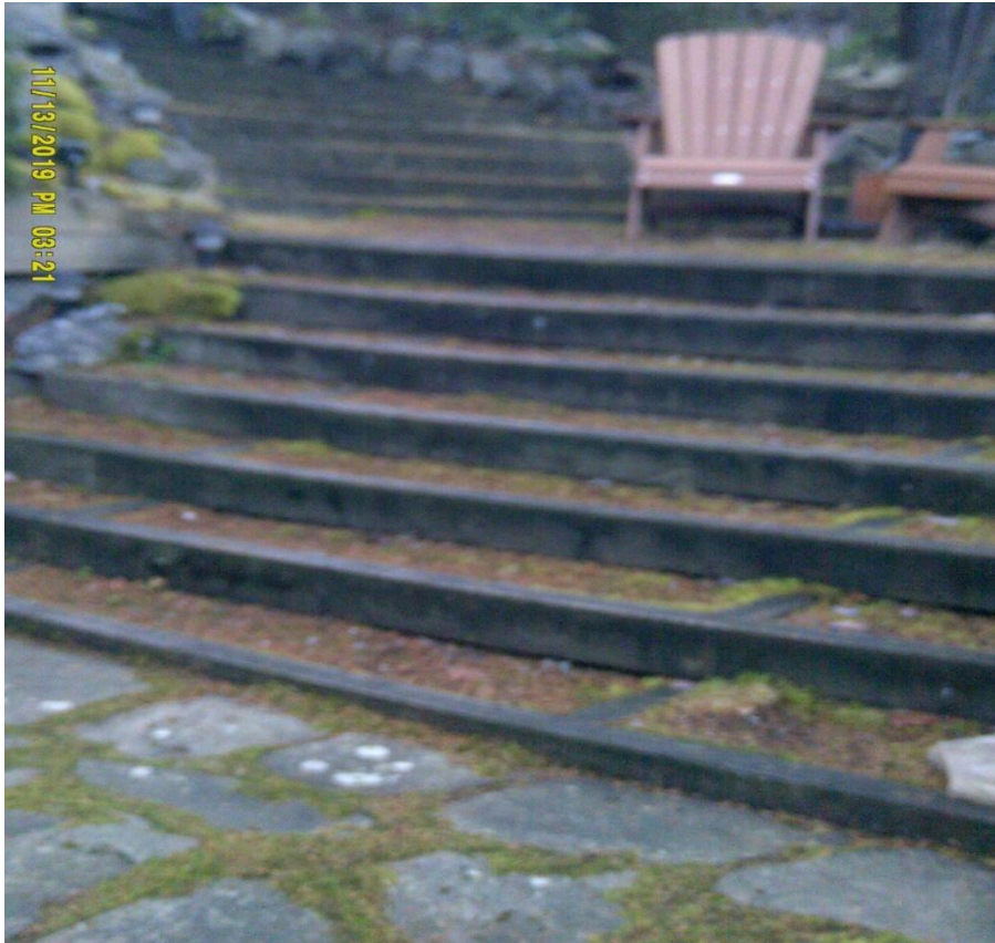
PHOTO 3.6 (IN) Stairs to enter home
