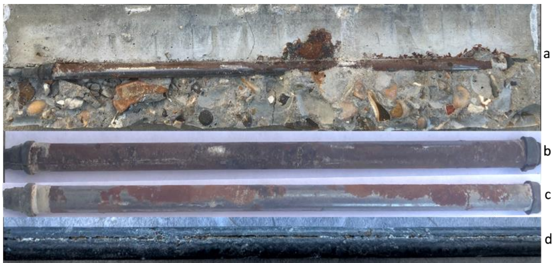
Fig. 6.18 The amount of rust formed on the surface of the rebar in specimen type C made of FA: (a) the visual appearance of the specimens after the splitting into halves along the crack; (b) the surface of the rebar facing the crack, (c) the side away from the crack (d) the surface of the bar facing the crack after the picking.
