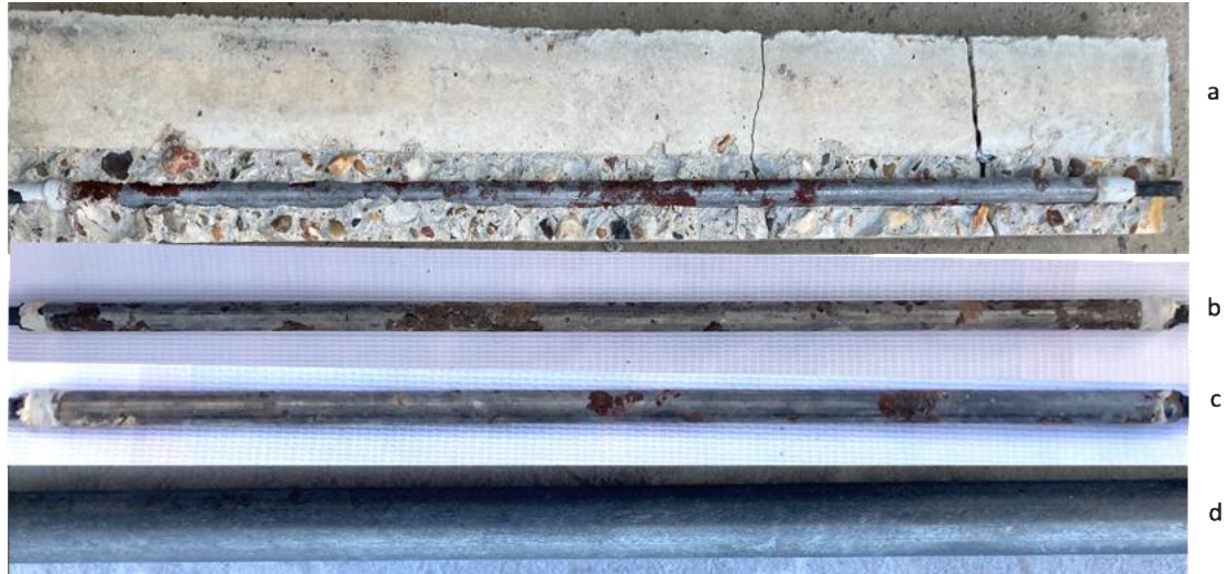
Fig. 6.11 The amount of rust formed on the surface of the rebar in specimen type B made of GGBS: (a) the visual appearance of the specimens after the splitting into halves; (b) the surface of the rebar facing the crack, (c) the side away from the crack (d) the surface of the bar facing the crack after the picking.
