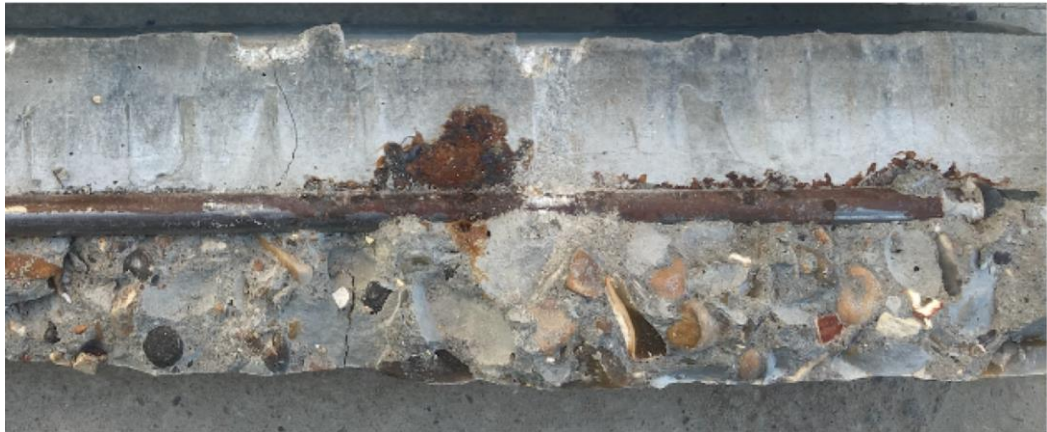
Fig. 5.15 Crack-steel interface in the artificially created crack that reaches the rebar level, specimen type C.
