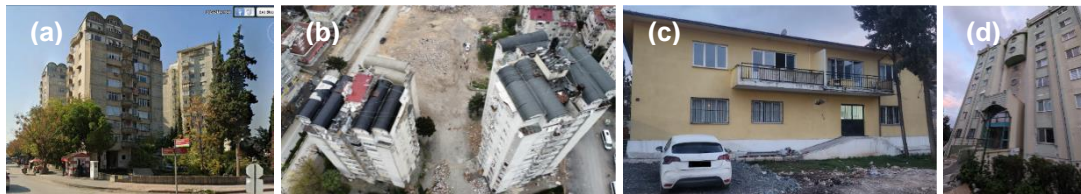
Figure 7: (a) 3-building complex before (b) and after the earthquake; (c) Masonry building with carbon-fibre-reinforced polymer retrofit; (d) TOKI building with minor damage.
