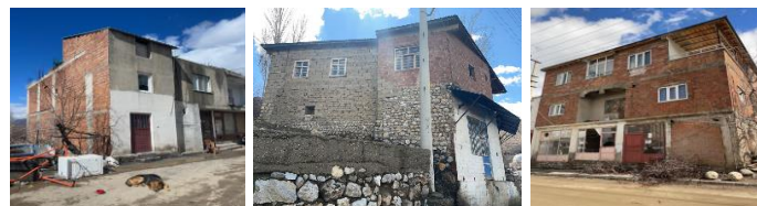
Figure 6: Examples of non-engineered buildings
