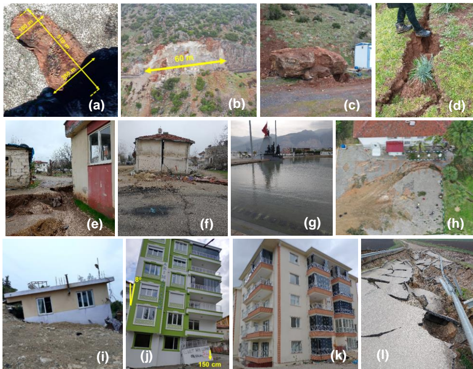
Figure 2. Geotechnical observations from the EEFIT mission (a) Landslide upstream of Değirmencik, (b) Landslide north of Türkbahçe blocking the rail line (c) Rockfall north of Türkbahçe hitting both an electricity tower and a water line (d) Surface rupture on a hill (e) Interaction of surface crack with a stiff, strong foundation (f) Interaction of surface crack with a weak foundation (g) İskenderun Anıt Meydanı square subsidence (h) Lateral spreading at the school of Demirköprü (i) Shallow-founded structure at an area of liquefaction (j) Building with a shallow foundation and high aspect ratio in Gölbaşı (k) Building with a shallow foundation and low aspect ratio in Gölbaşı, and (l) Embankment failure close to Çöçelli
