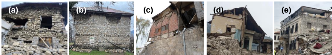
Figure 5: (a) URM (separation wall-leaf); (b) timber reinforced stone masonry (arch failure); (c) Himiş (OOP of bearing wall), (d) gable failure, and (e) addition of a storey
