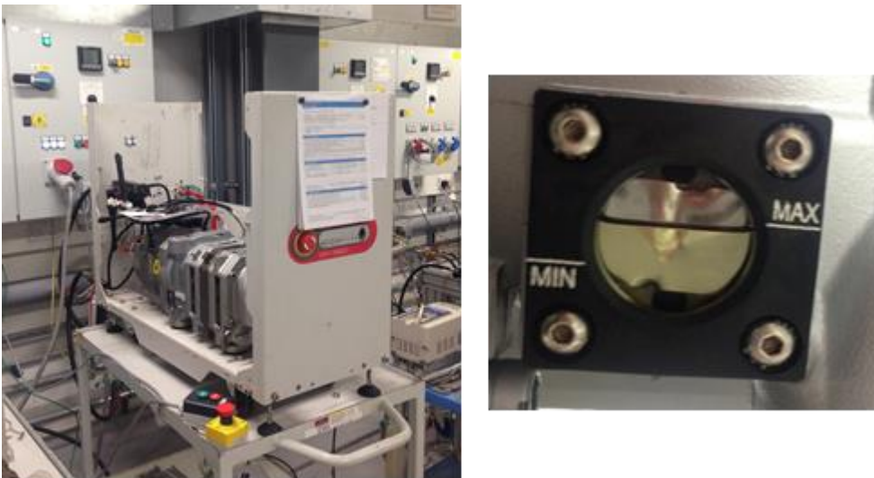
Figure 38 Pump ready to be started on left, right with indicator showing the correct amount of lubricant has been added
