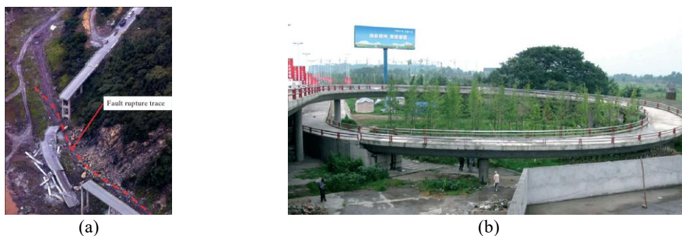
Fig. 1. Seismic damage of curved bridge during the 2008 Wenchuan earthquake: (a) Baihua Bridge; (b) Southeast ramp of Huilan interchange.
