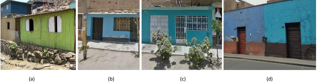
Figure 2: Building types categorised by construction (thermal mass) in José Carlos Mariátegui and Barrios Altos. (a)Light (b)Medium (c)Heavy (d)Traditional
