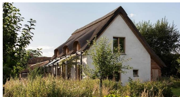
Fig. 1. Case study building, east elevation [2]
