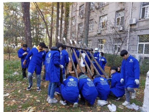
(b) Lifting the right wing of the bridge
