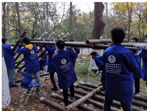
(c) Placing the top of the bridge
