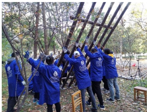
(a) Lifting the left wing of the bridge
