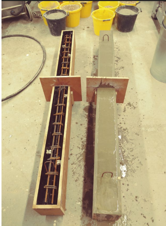
Fig. 3: Beam concrete casting
