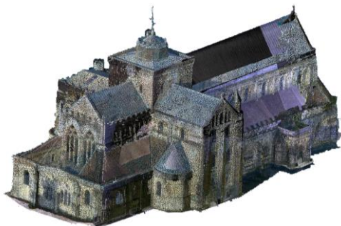
Figure 3. Registered point cloud from Romsey Abbey.
