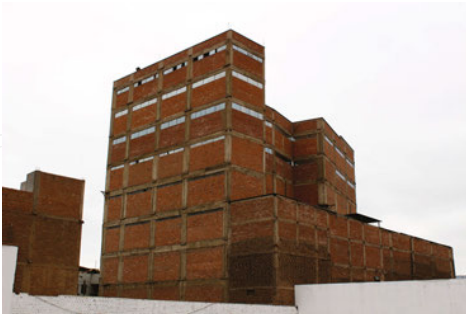
Figure 2. The storage facilities that violate the building height restrictions for the historic centre and come to replace the old structures within an area deemed of monumental value. Source: Photo by Rita Lambert.
