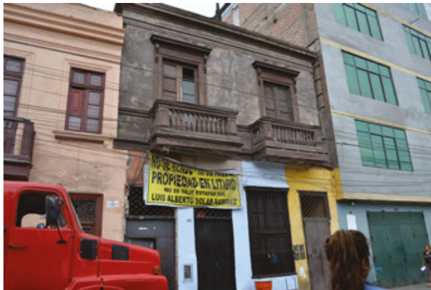
Figure 1. A building in Barrios Altos marked as ‘Property under litigation’, a sign that illustrates the disputes and conflict with land traffickers posing as owners. Source: Photo by Rita Lambert.
