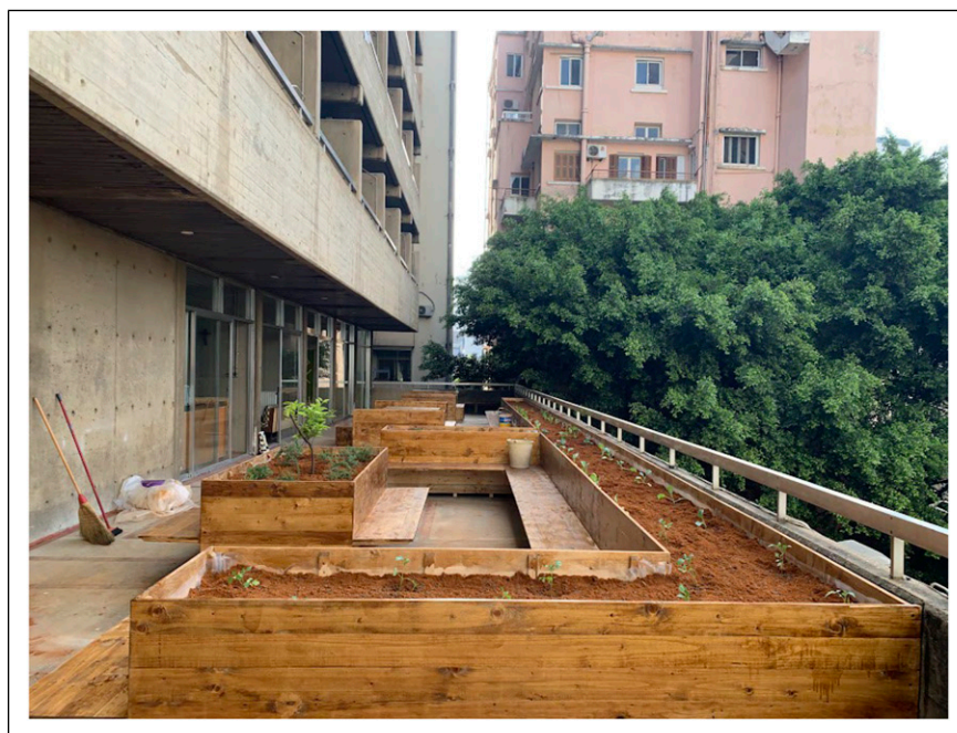
Figure 9. The intervention after completion.
