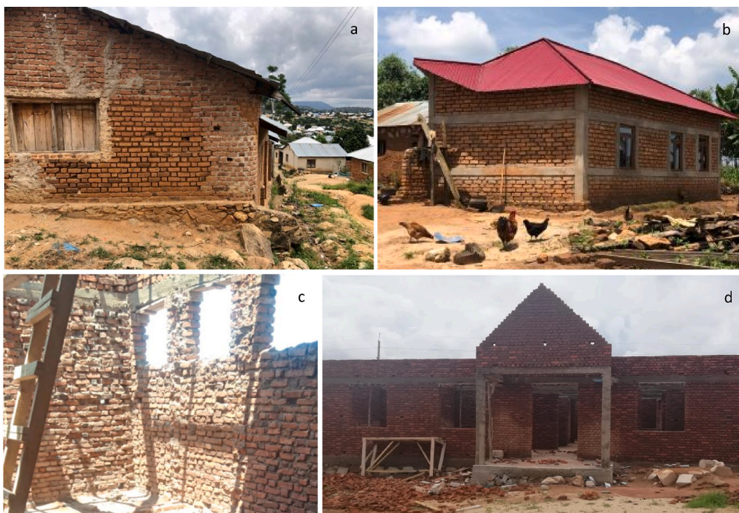
Fig. 3. The local built environment: (a) typical unreinforced burnt bricks masonry dwelling; (b) building with rare RCC horizontal and vertical bands, which are an optimal seismic detail; (c) and (d) unreinforced burnt brick masonry building under construction. (Iringa, 2021).
