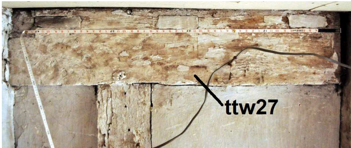
Figure 11: The girthing beam in truss 14 sampled for dendrochronology (photograph Duncan James)
