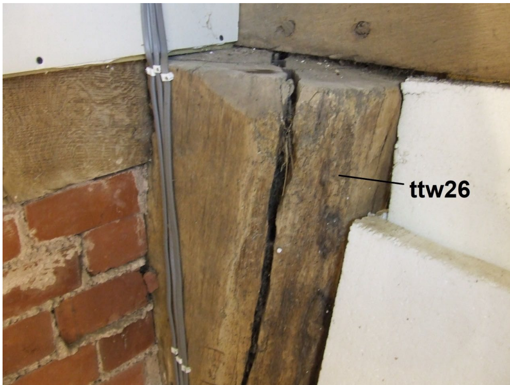
Figure 10: View of the west post of truss 15 sampled for dendrochronology (photograph Martin Bridge)
