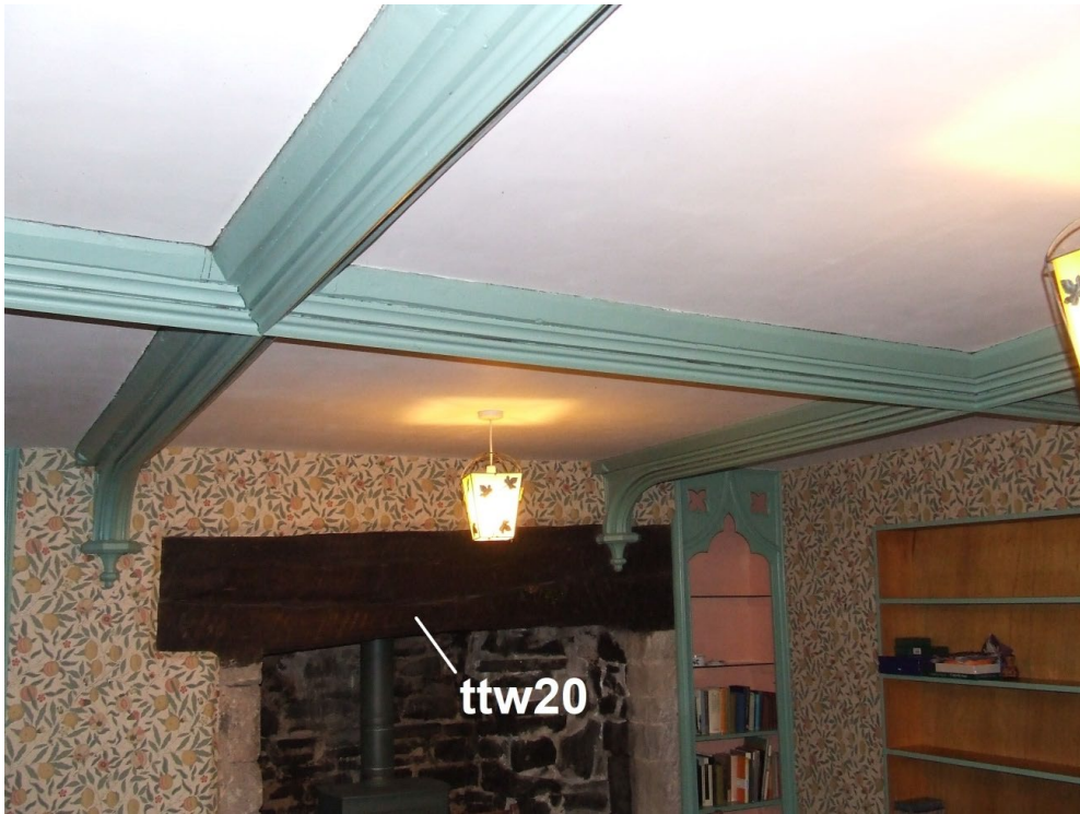
Figure 9: Ground floor of bay 5, showing the fireplace lintel sampled for dendrochronology (photograph Martin Bridge)
