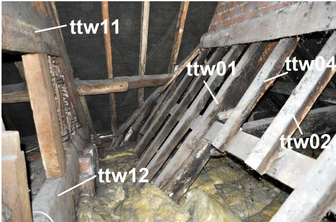
Figure 5: View of the south side of bay 1 on the right, with truss 8 on the left, showing timbers sampled for dendrochronology (photograph Duncan James)
