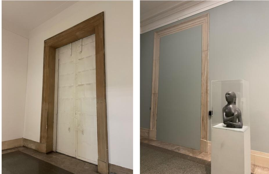
Figure 7.3: Blocked connections between the central axis and the east side
