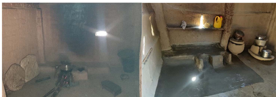
Figure 6. Holes in the wall for ventilation. Source: Authors' TEG cookstove survey, 2021.
