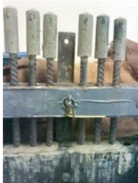
(d) Casting mortar on top of the self-amalgamating tape at the other end
