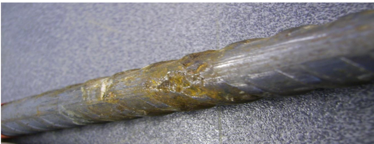
(a) AAS - corrosion evident on the highlighted area surrounded by sound regions, localised pitting evident
