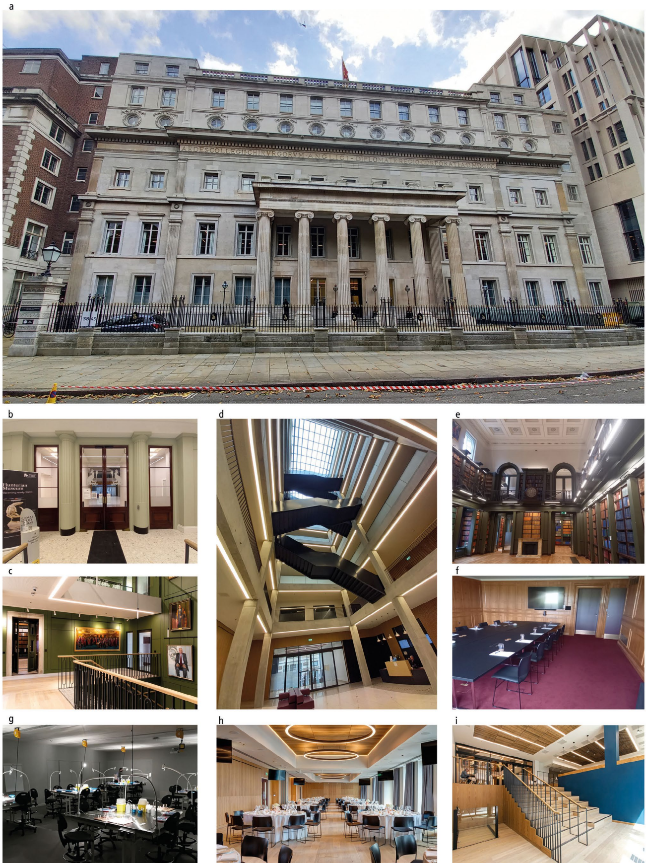
Fig. 1 a, b, c, d, e, f, g, h, i) The newly refurbished Royal College of Surgeons of England building in Lincoln's Inn Fields, Central London. The frontage of the original building has been retained, while the front and rear entrances have been redesigned. The interior space is dominated by a light and expansive atrium traversed by the main staircase, the original library has been restored and refurbished, and there are numerous state-of-the-art teaching areas, meeting rooms and conference facilities. The Hunterian museum is currently being redeveloped and is due to open in early 2023
