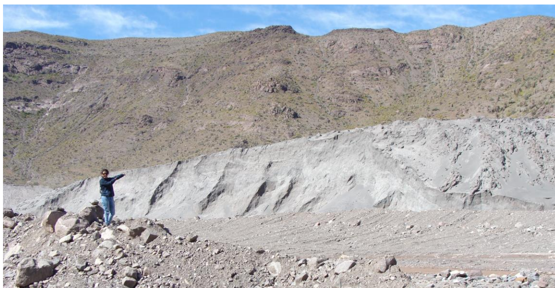
Figure 3 Eroded section of tailings deposit 3 (Figure 2) in the Marquesa valley photographed in September 2017 and showing the steep slope left after failure, which reveals internal stratification of tailings
