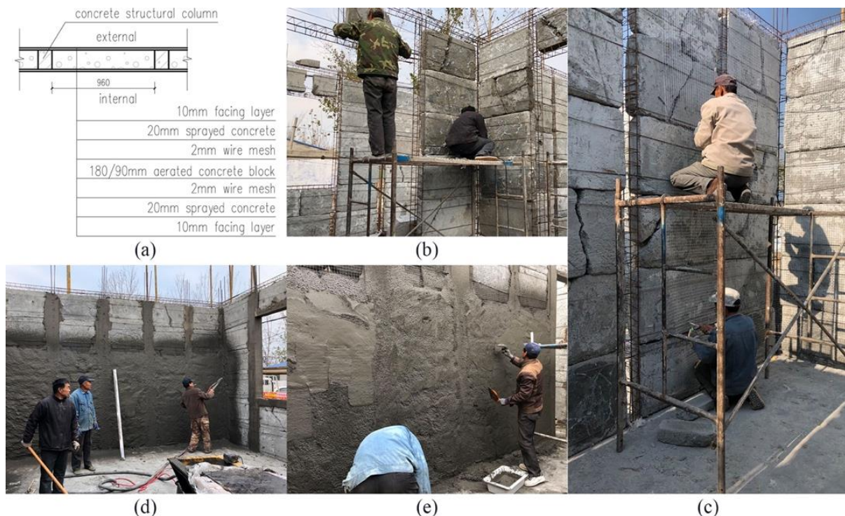
Figure 3. Design details (a) and construction process (b-e) of the wall
