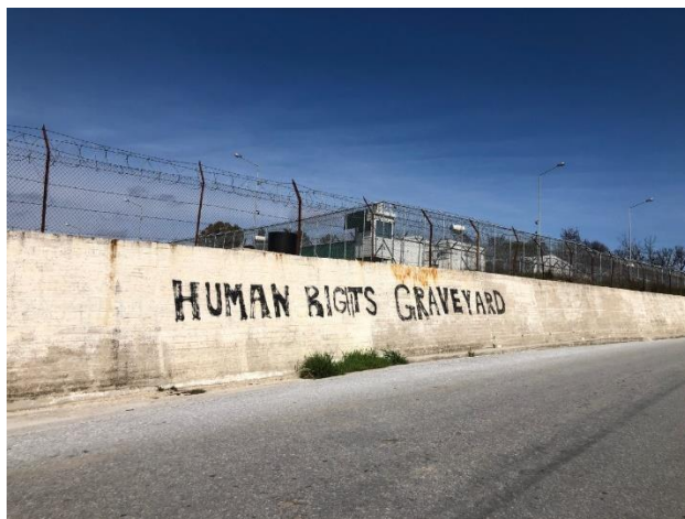
Figure 1: Boundary wall of Mória Refugee Camp in Lesvos
