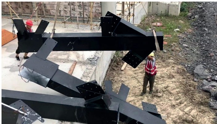
Figure 19.4a Onsite assembly: Connection steel components
