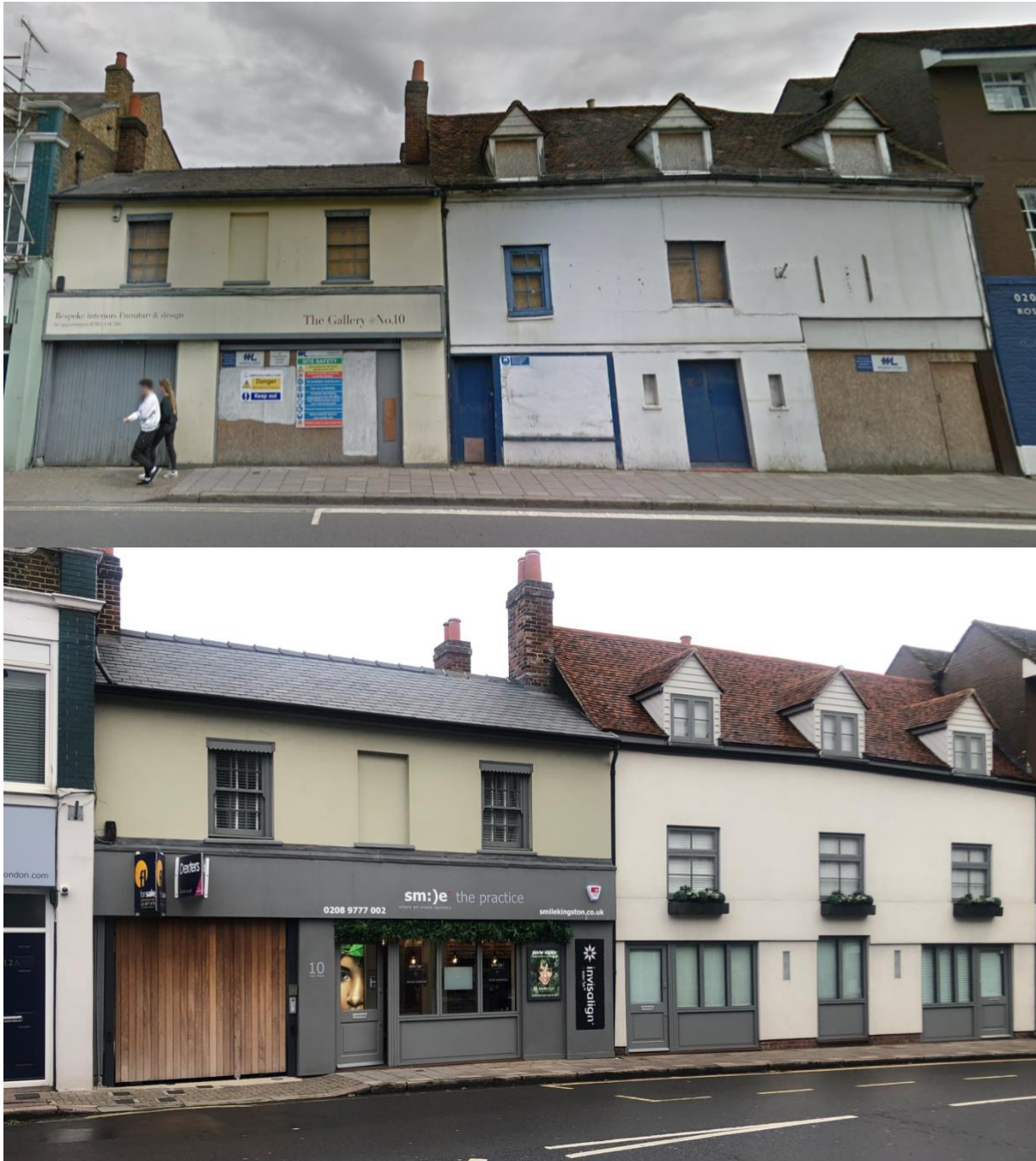
Figure 5 – 6-10 High Street, Hampton Wick before and after conversion to residential use (top photo from 2016 © Google and bottom photo from 2019 © Ben Clifford)
