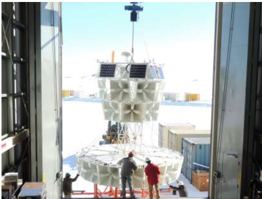
(e) The middle ring antennas are mounted. After this, the bottom ring of the gondola is constructed, and the final antennas and solar panels are attached.
