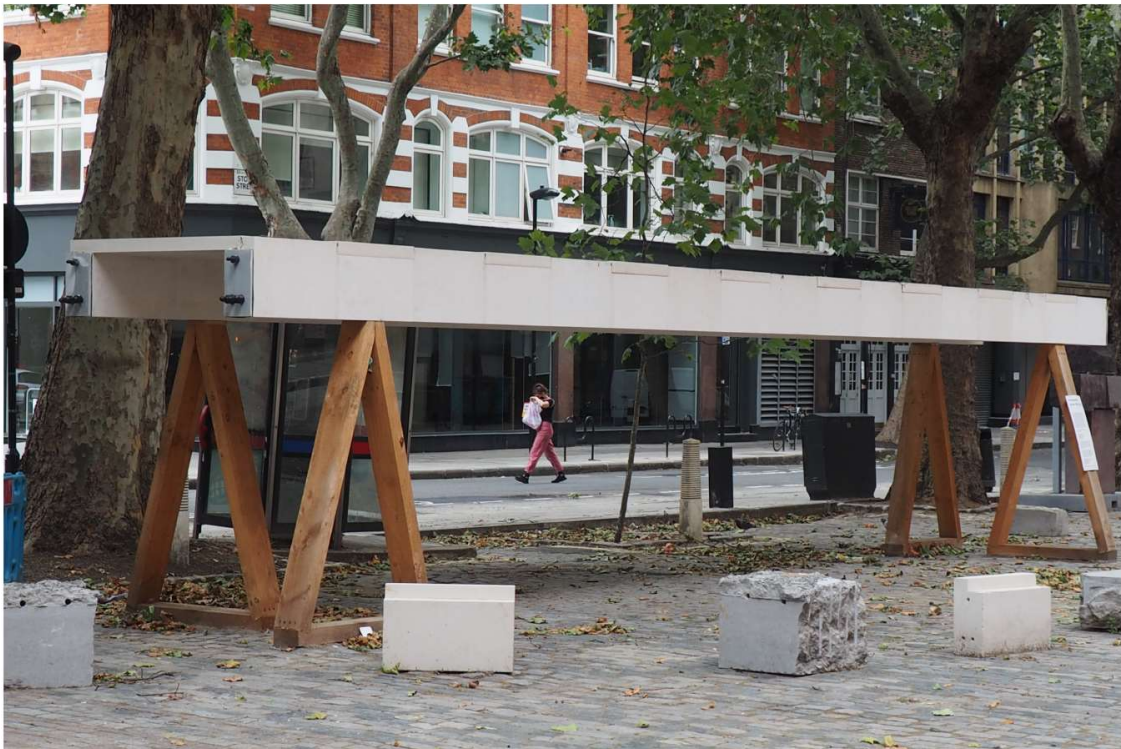
(a) 12 m Long Post-tensioned Limestone Floor Beams
