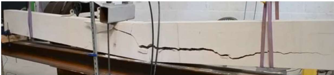
(b) Asymmetric failure crack trajectory
