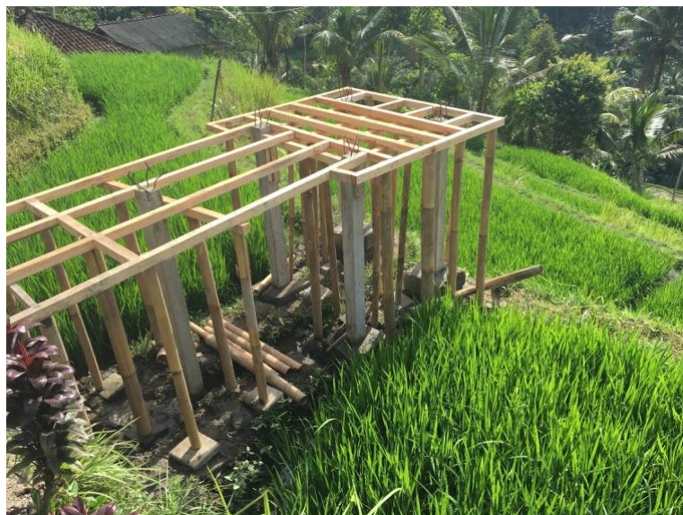
Figure 8-5. A development within Subak Pakerisan Watershed (Source: D. Rahman, May 2018)
