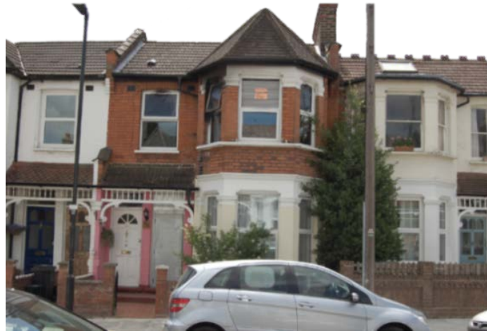
Figure 5: Front View of Hawthorn road house Source: Prestia (2010)
