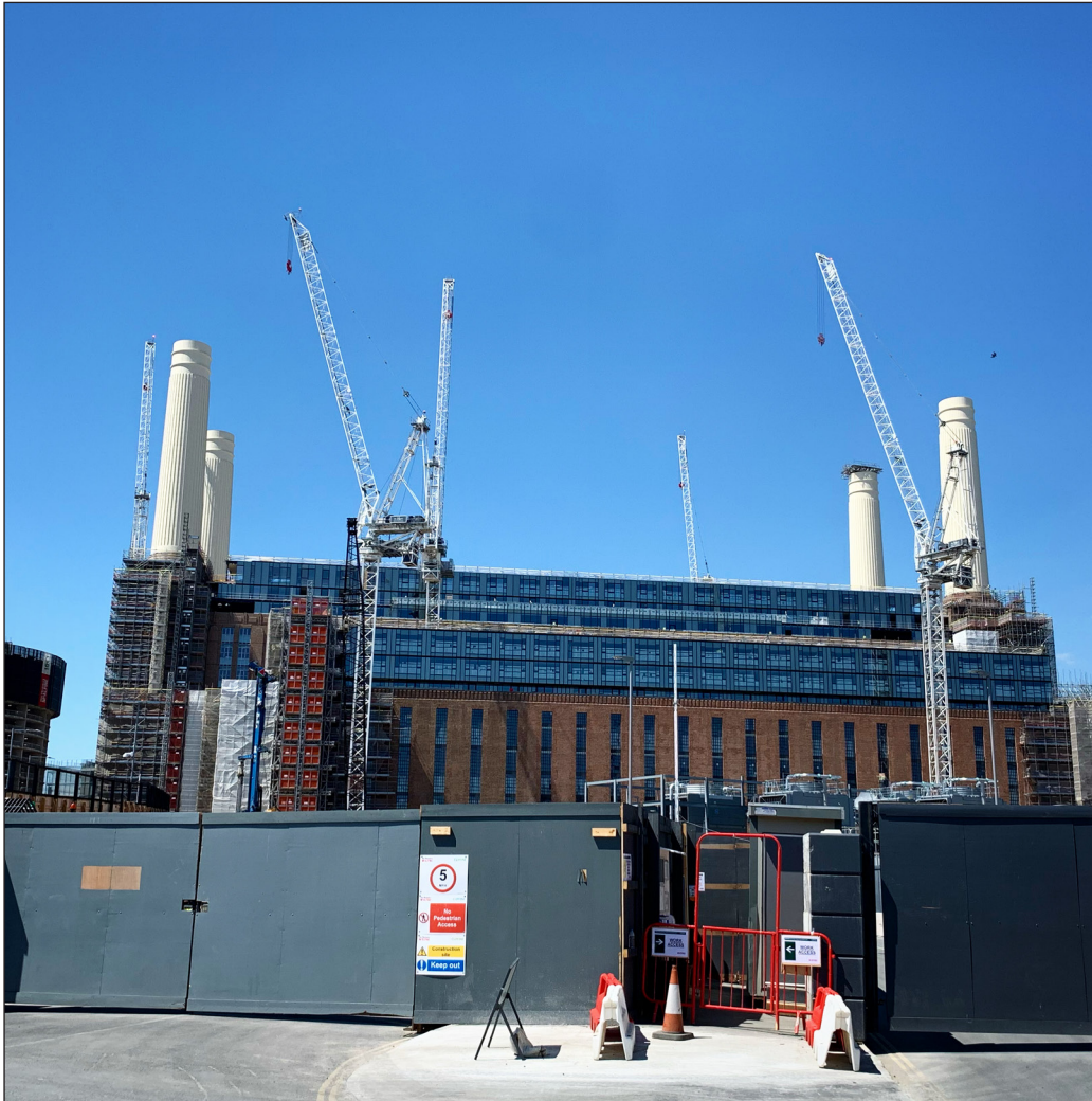
Figure 2: Battersea Power Station Redevelopment, Nine Elms.
