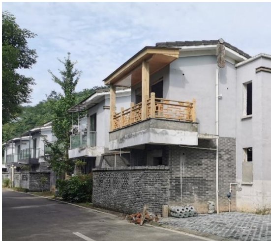
Figure 3: House under renovation
