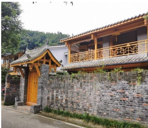
Figure 5: First-phase second home
