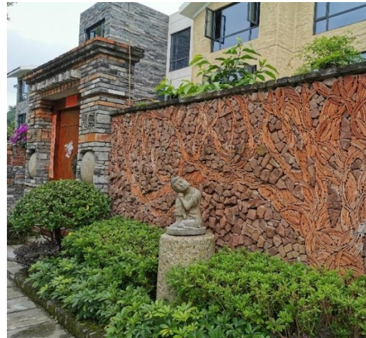
Figure 4: Façade of the second home
