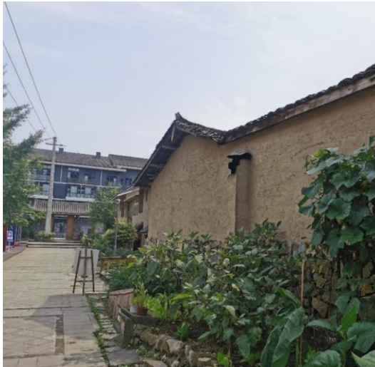
Figure 9: Traditional yellow clay wall of a resident's house
