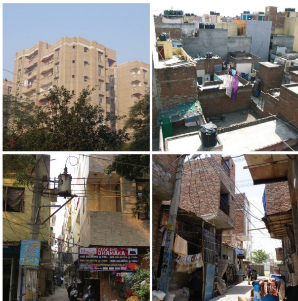
Figure 2. Examples of category 1: planned housing (top left), category 2: urban/rural villages (top right), category 3: unauthorised housing (bottom left), and category 4: JJ Clusters (bottom right).
