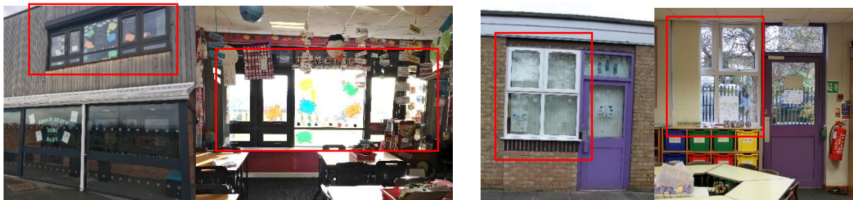
Fig 8. Classrooms with single-sided openings at two different sizes (outside and inside). Fig 9. Classroom with single-sided openings at one size (outside and inside)
