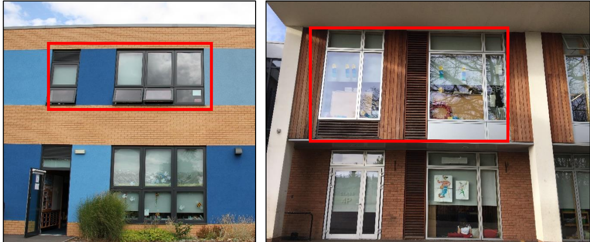
Fig 10. A classroom in school 1 providing louvre openings alongside windows. Fig 11. A classroom in school 6 providing louvre openings alongside windows
