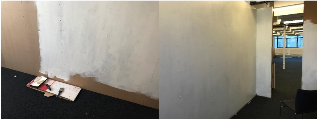
Figure 7- 10: Surface refurbishment in progress
