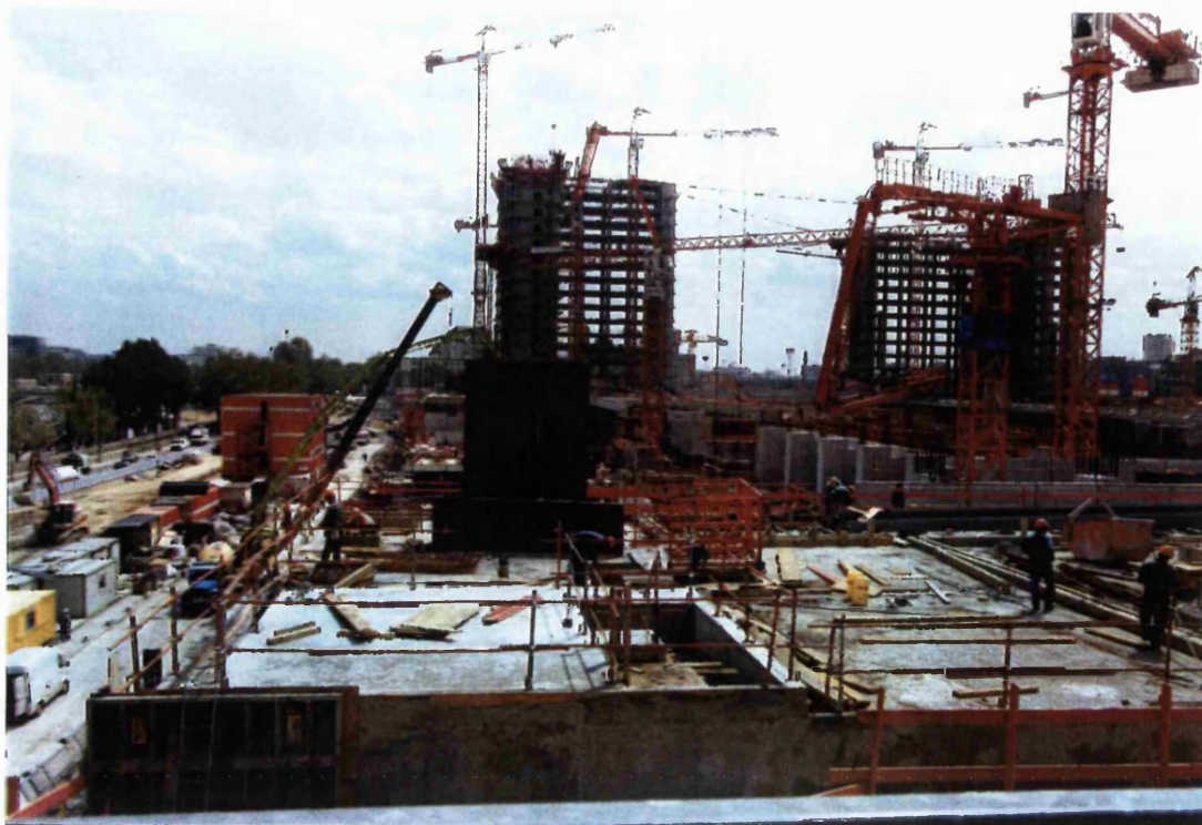
Fig. 9.98: Work progress on site, April 23, 1993
