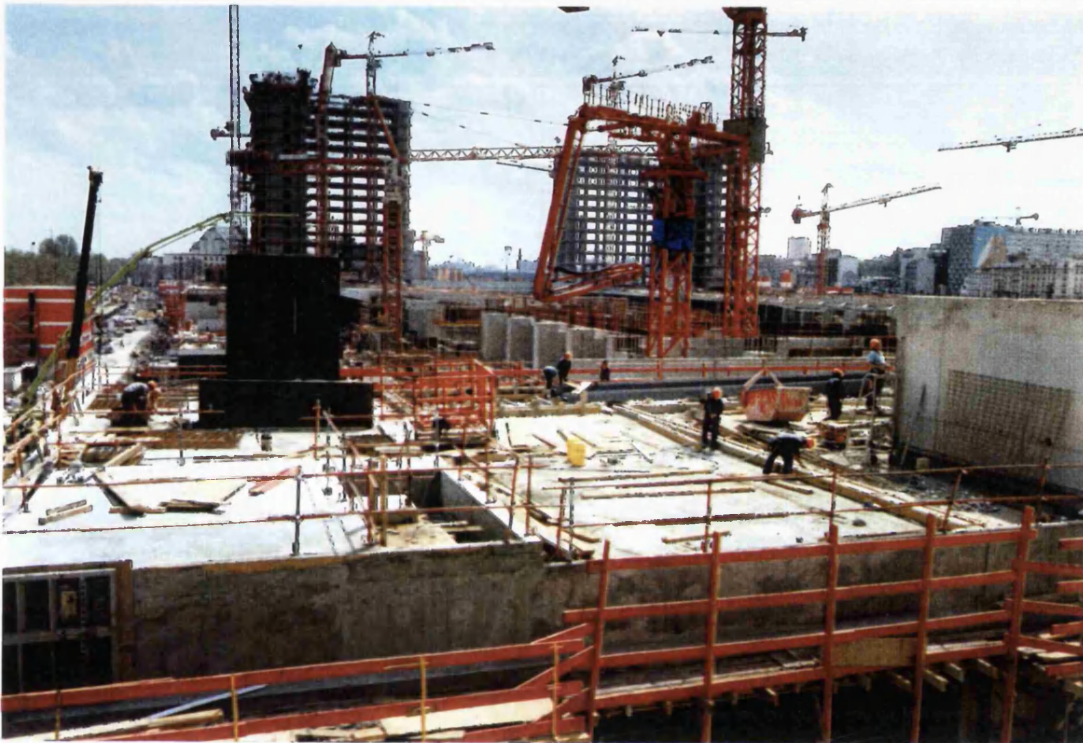
Fig. 9.91: Work progress on the Bibliothèque (April 1993)
