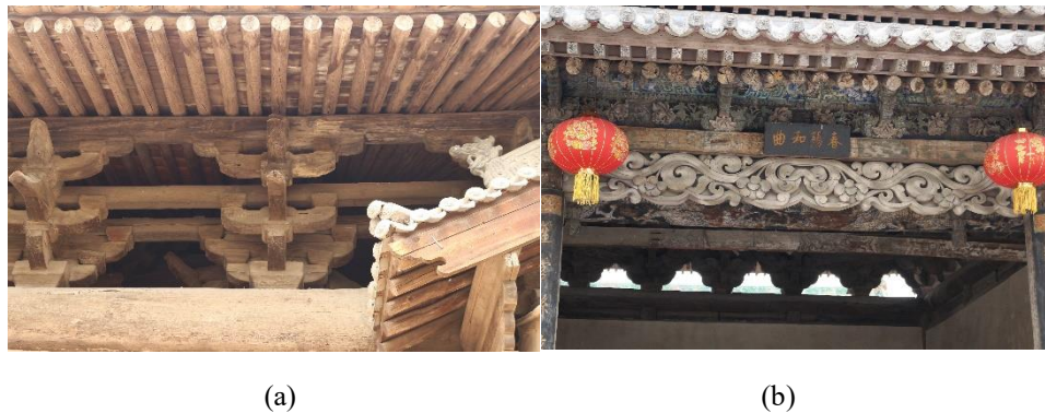
Fig. 2 Photographs of ‘brackets’ of the traditional Chinese buildings, (a) ‘brackets’ of the Yuan dynasty, (b) ‘brackets’ of the Ming dynasty
