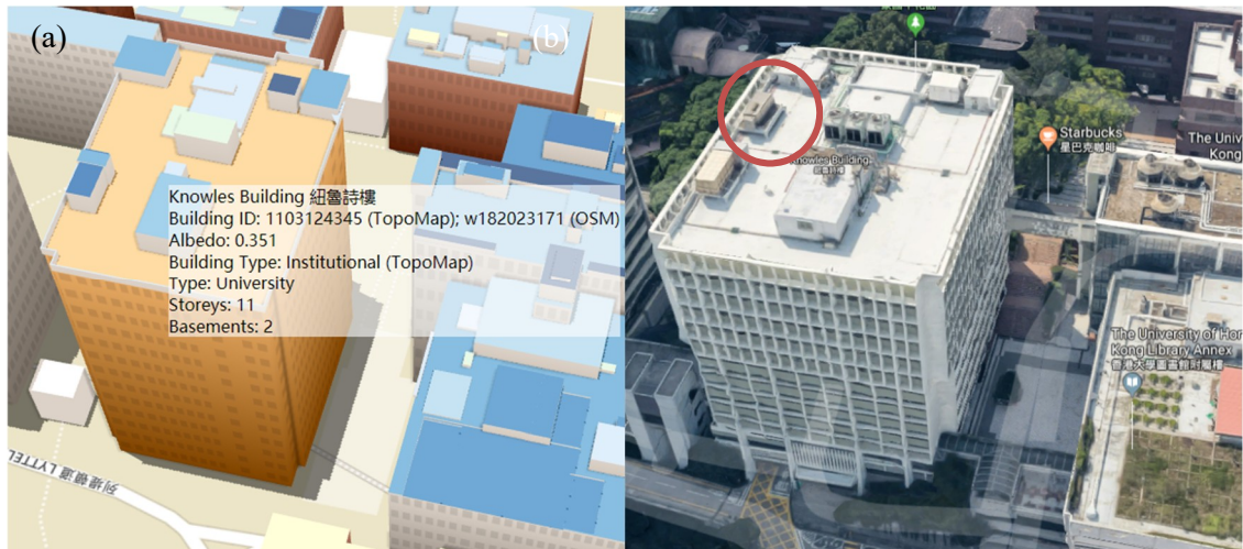
Figure 4. Example of the output model. (a) Roof and rooftop elements of Knowles Building, HKU (cooler color indicates higher albedo), (b) the referential 3D building model in Google Earth, where the circled is a missing element in (a).
