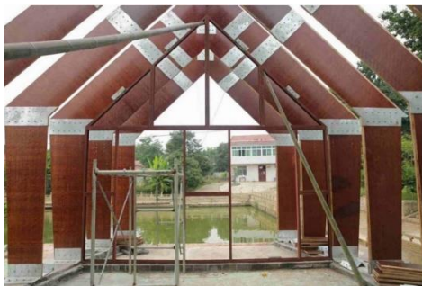
(a) Under construction
