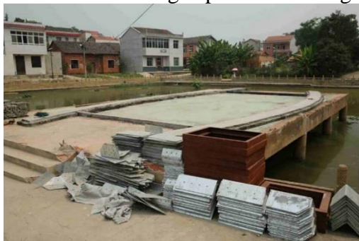
(a) On-site material placement
