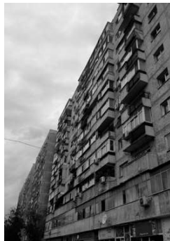
Urban housing corridor. Bucharest, Romania. Photo: Iulia Statica, 2013.
