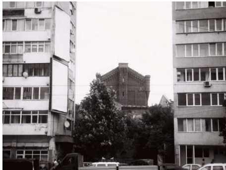
Industrial space behind communist housing blocks. Bucharest, Romania. Photo: Iulia Statica, 2014.
