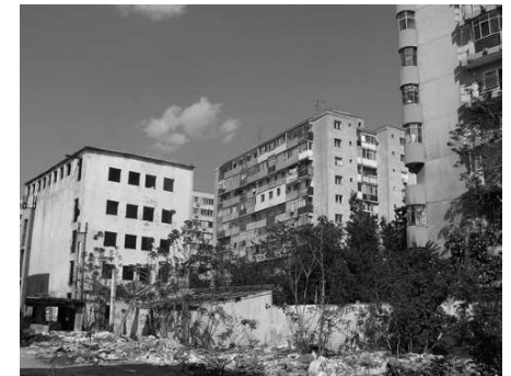
Industrial space behind communist housing blocks. Bucharest, Romania. Photo: Iulia Statica, 2013.
